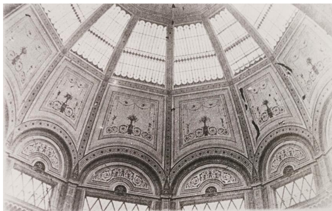
Image 4: The first Alexandra Palace re-used materials from the 1862 International Exhibition. This is the dome roof of the first Palace. 5
